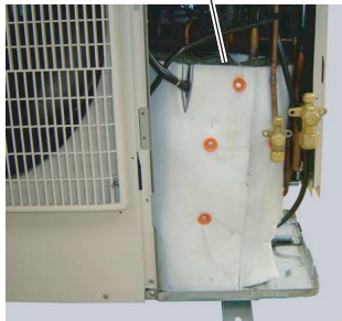
Remove the COMPRESSOR COVER BODY and TOP.
