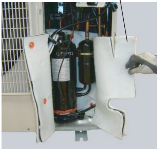
Remove the COMPRESSOR COVER BODY and TOP.
